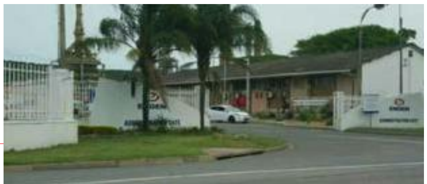
The current ATR main entrance in Wentworth (2007) after being taken over by Engen Refinery. The brown building used to be the Chemistry laboratory where all first-year medical students were taught by the infamous Mr Paris, who was feared by most if not all first-year students.
