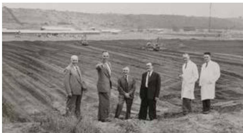
The students' sport field in construction in the foreground and the ATR in the background, March 1953.
